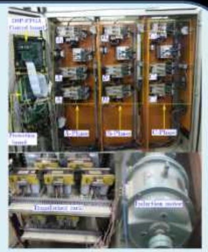
Cascaded H-Bridge Inverter Drive
